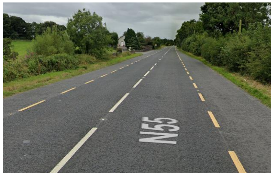
Figure 3-15 National road N55 at Annagh Lower Invalid source specified.
